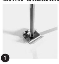
Fix clips with suitable screws (min. 2 per metre/40"). Drill cable hole/s if required.
