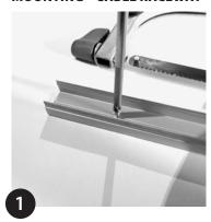
Cut raceway to desired length. Drill holes to suit screws and fix in place. Drill cable holes if required.
